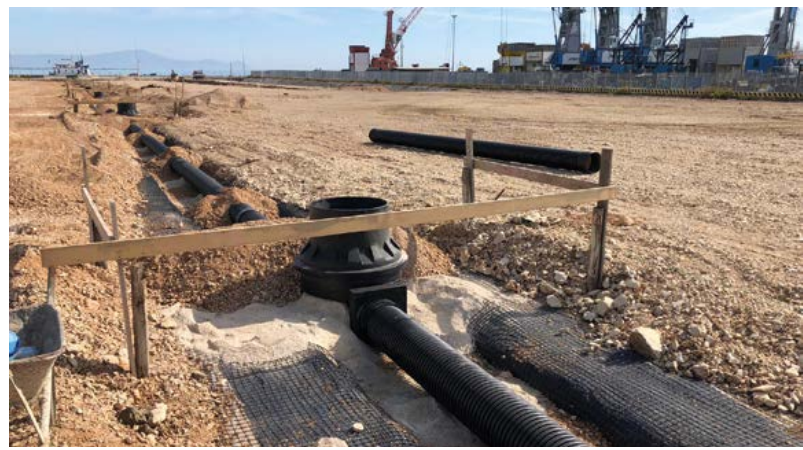
Formed manholes Ø1000 - Salerno (SA)
