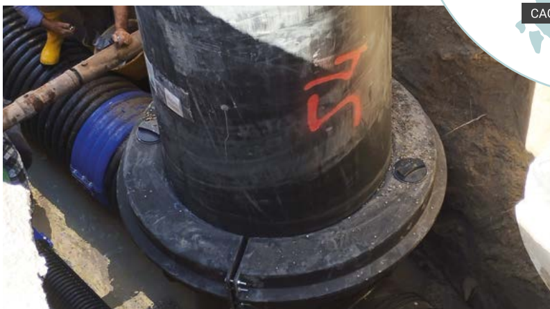
Formed manholes anti-layer Ø1000 - Cagliari (CA)
