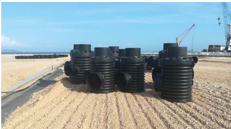
Formed manholes Ø1000 - Napoli (NA)
