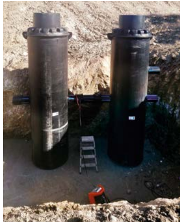
Formed Manhole Ø1000 - Chieti (CH)
