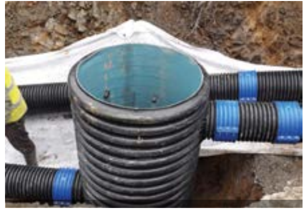
REALIZATION OF DRAINAGE SYSTEM WITH TAILOR-MADE CASCADE MANHOLES
