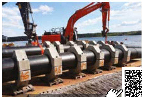
STOCKHOLM (SWEDEN 2019): PRESSURE SEWERAGE SYSTEM FOR SUBMARINE CHANNEL CROSSING IN THE CITY
