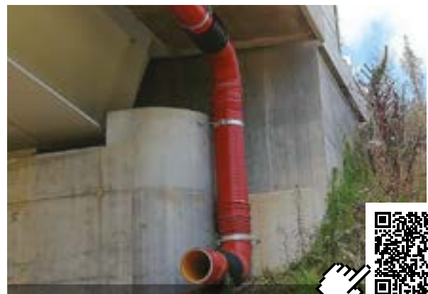
BOLOGNA (ITALY 2019): NEW BRIDGE DRAINAGE SYSTEM
