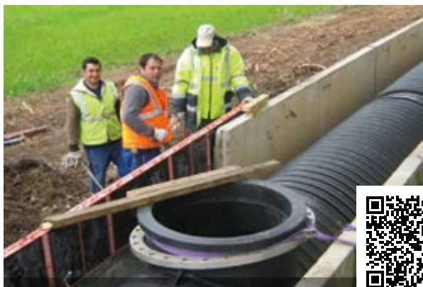
FLORENSAC (FRANCE 2009): DAMAGED CONCRETE CHANNEL REHABILITATION WITH PIPE INSERTION
