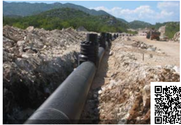
CROATIA 2006: STORM WATERS DRAINAGE SYSTEM CONSTRUCTION FOR A NEW MOTORWAY
