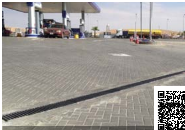
JERASH (JORDAN 2016): RAINWATER DRAINAGE CHANNELS REPLACEMENT IN SERVICE STATIONS
