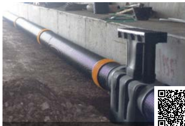
RICCIONE (ITALY 2012): NO-FIRE SYSTEM FOR ENVIRONMENTAL PROTECTION AND ANTI-SPREAD OF FIRE IN THE COLLECTOR OF THE ROAD TUNNEL
